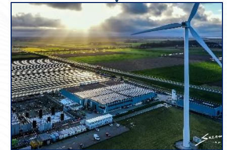
Start construction Phase 2A
